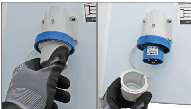
Opening the mains connection
