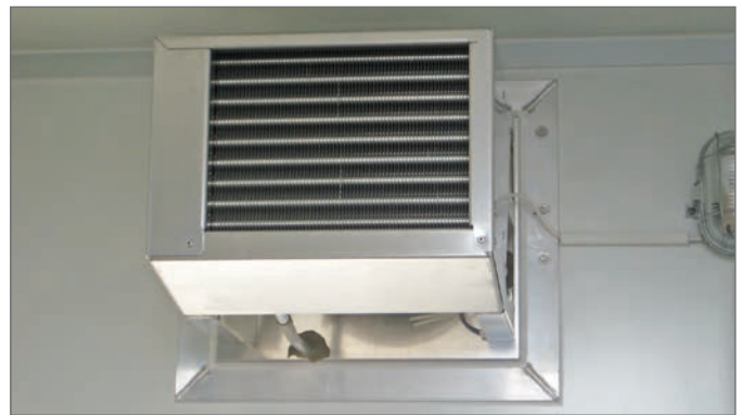
Internal view of HCU
