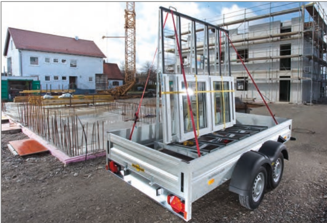
Secured with tie-down
