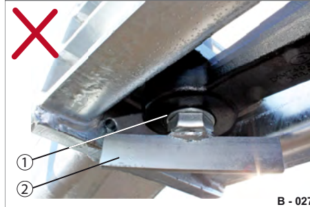
Fig. 26 Incorrectly secured - view, bottom
