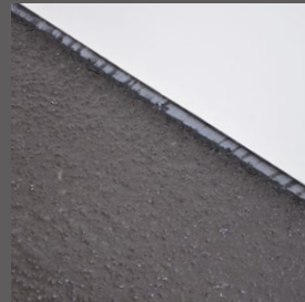
Flowing screed floor
