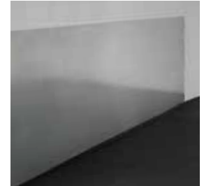
Side kick plate made of sheet metal
