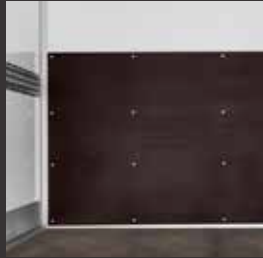
Front wall reinforcement
